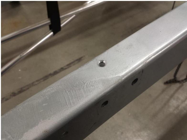
Figuur e: Drilled hole for the sensor cable
